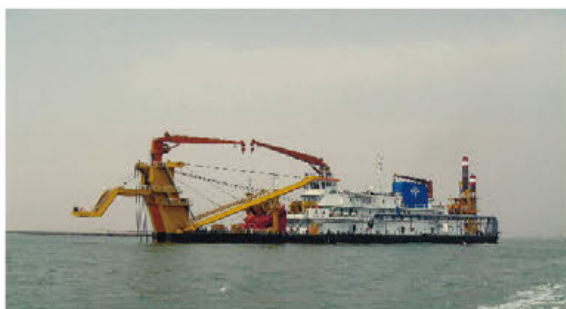
中交天津航道局天骥号挖泥船作业现 “Tianji” Dredger Of CCCC Tianjin Dredging Company Working On Site
