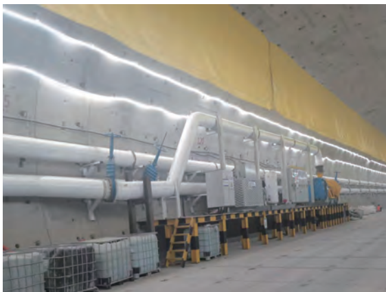
中铁隧道上海机场线 China Railway Tunnel Shanghai Airport Line
