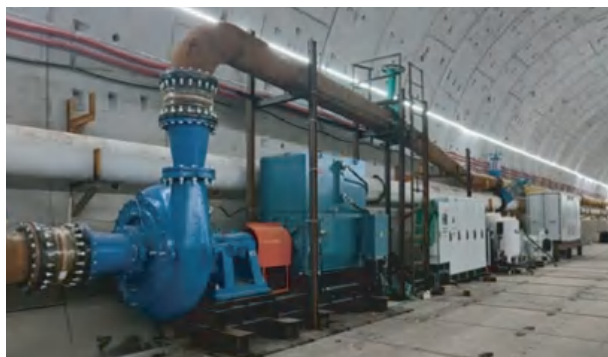
Shanghai Infrastructure 15m Tunnel Project
