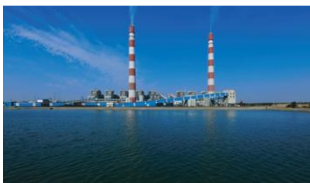
India Jharsuguda Power Plant Desulfurization Project
