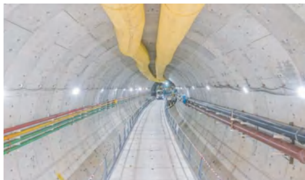
China Railway 15th Bureau Hengqin Project
