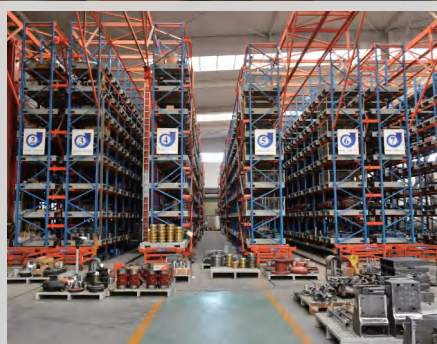
Automated Storage & Retrieval System (AS/RS) Warehouse
